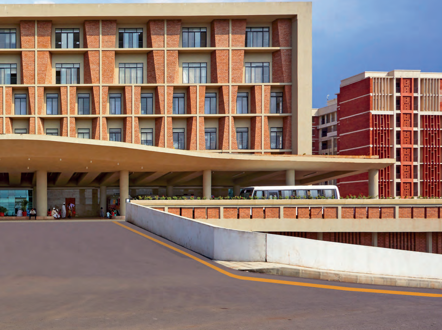
Entrance porch at SUHRC.
